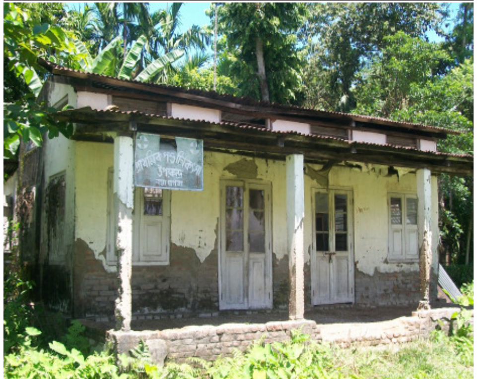
The dilapidated condition of Veterinary Sub-Centre at Naya Gogra in Chengaigaon clearly reflects apathy on part of administration and the State Government. Picture courtesy- Tanushree Hazarika
